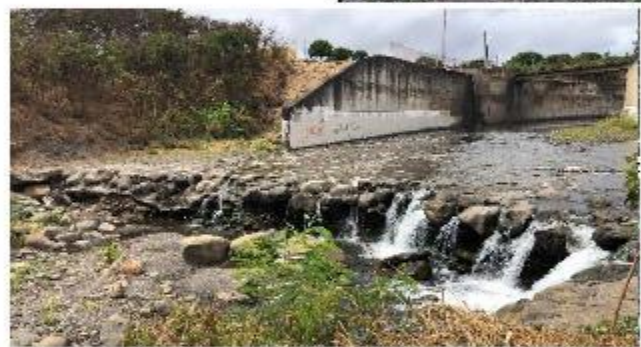
Existing head cut at upstream lined channel; proposed location of pre-formed scour hole
